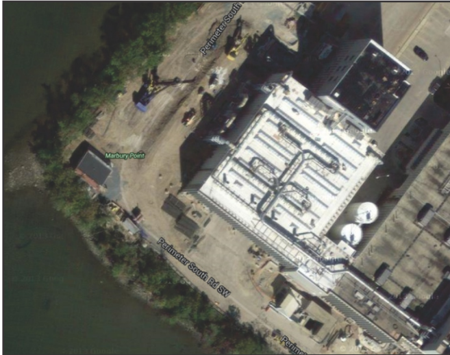
Aerial view of dewatering facility showing PSP ® duct on the roof.
