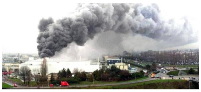
Building loss in excess of \$400 million USD, exclusive of production and downstream interdependency losses. A contributing factor to the spread of the fire was the use of plastic exhaust duct.
